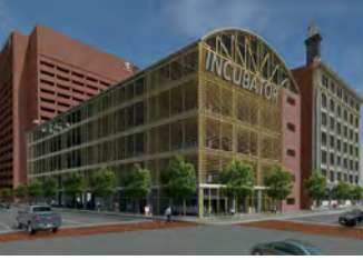
Incubator & Arts Academy UTA - Adolfo Gonzales Left above, shared Office Incubator for Techies and Startups features truss roof, stick built structure over concrete garage to replace existing parking; Right above, Re-Use of vacant Entertainment Center as Arts Academy features Media Board visible from adjacent freeway.
